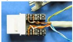
**4** Punch down the remaining pairs. Avoid damaging the wires with the punch-down tool.
