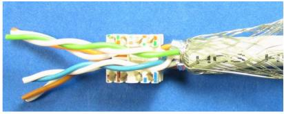
**5** Cut the wires flush with a sharp tool.
