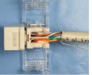
10 Wrap the drain-wire around the cable and close the metal shield.
