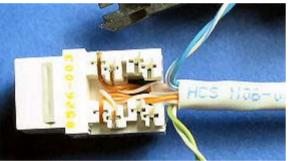
**4** Punch down the remaining pairs. Avoid damaging the wires with the punch-down tool.
