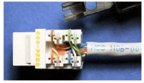
Notes: Keep the unjacketed portion of cable as short as possible. Keep the wires of each pair tightly twisted up to the point of termination. T568B pair/pin assignment is recommended.
