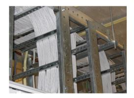
When CAT6 U/UTP LS0H cables are installed in large sites (as shown in the left picture) they must comply with IEC 60332-3. IEC 60332-1 cannot predict the performance of these cables under fire.
